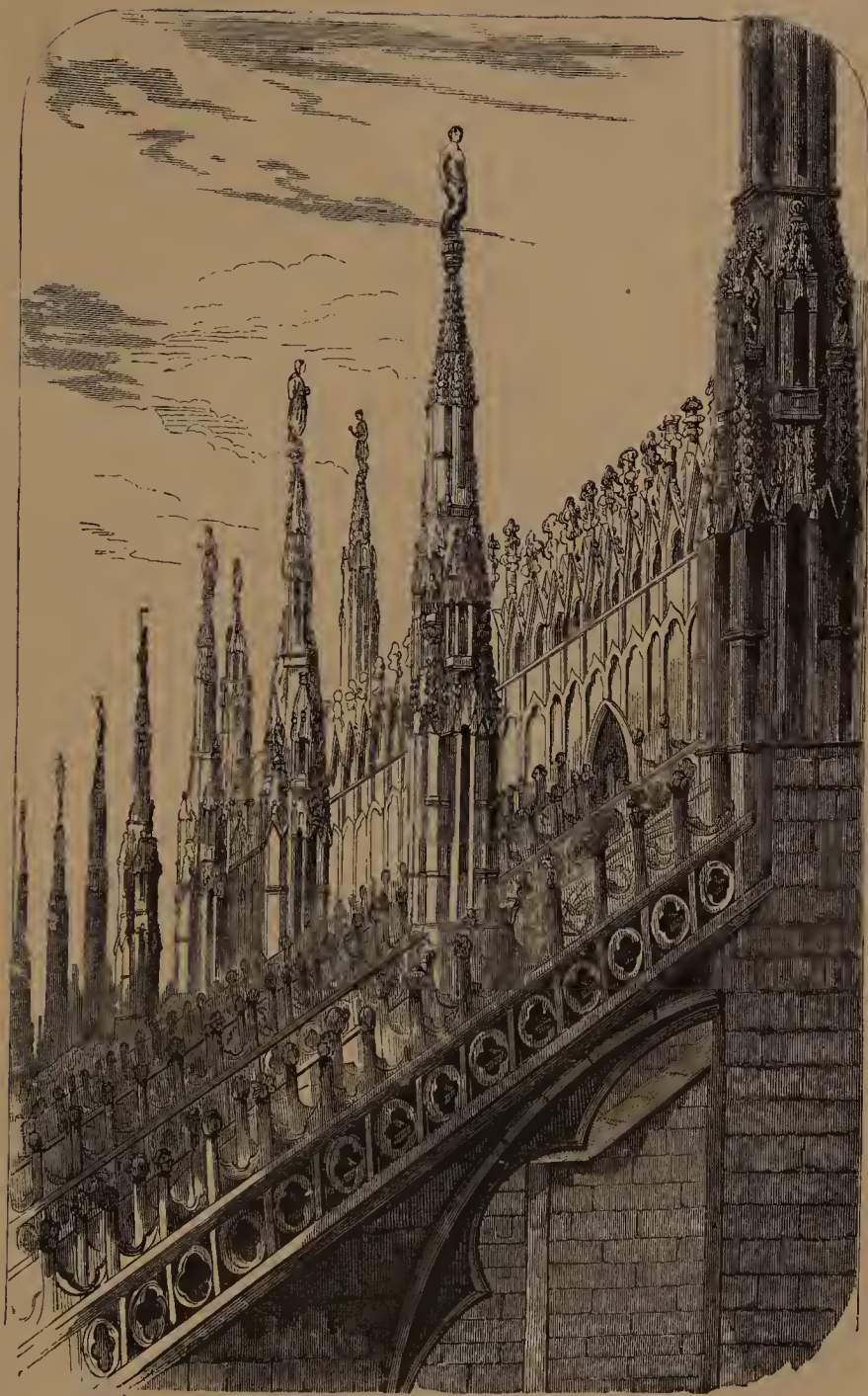
ROOFS AND SPIRES OF CATHEDRAL AT MILAN.
